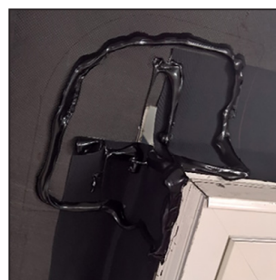
Fig 1. OT015 Adhesive beads applied; linear membrane already bonded
